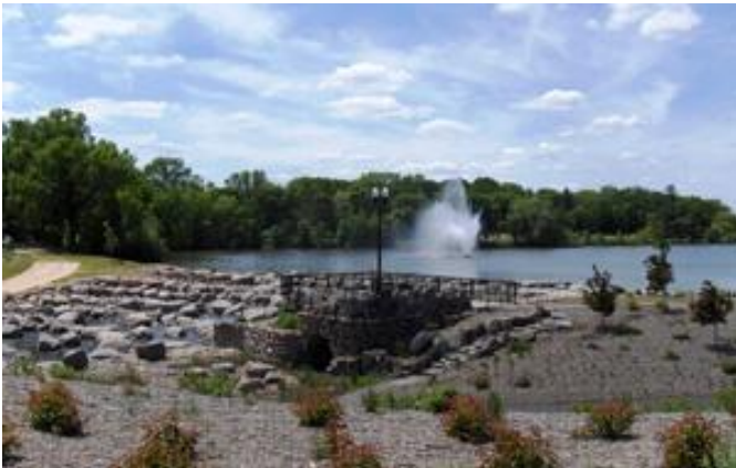
Newly Renovated Crow River Dam in Hutchinson
