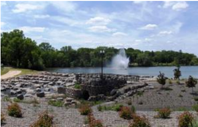
Newly Renovated Crow River Dam in Hutchinson
